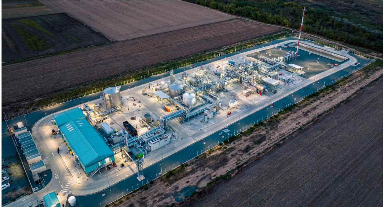
Image 4 Gas Treatment Plant in operation, September 2022
