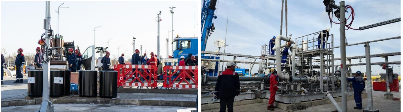
Image 1 and 2 GTP controlled shutdown, October 2023
